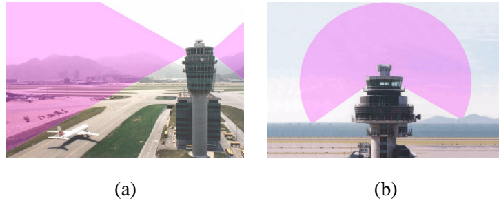
Fig. 1. Air traffic control tower. (a) FOV is limited by the supporting frame. An ideal case is to have a wide FOV as illustrated by the shaded region in (b).
